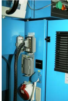
Example: PDDI mounted to control cabinet
